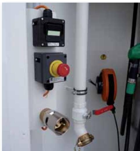
filling system filling pipe with tank vehicle connection, niche lighting switch, emergency stop switch and limiting-level transmitter (plug)
