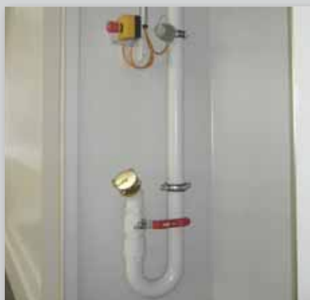
filling pipe, installed in dispensing niche
