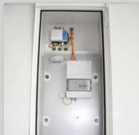
electrical niche with distributor
