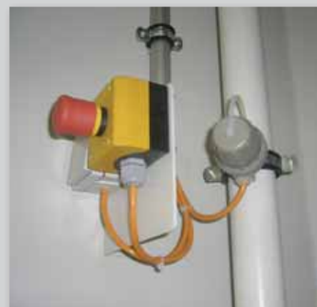
safety apparatuses: emergency stop switch, plug for limiting level transmitter
