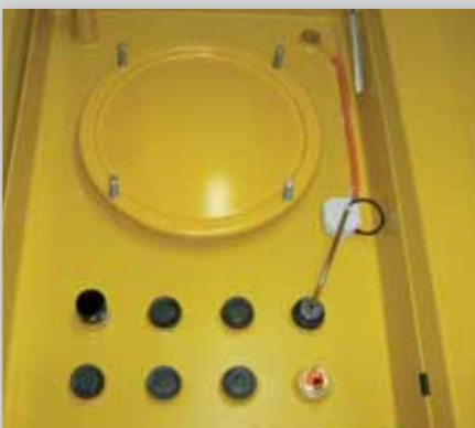
hatch compartment with dome cover, connecting sleeves, limiting level transmitter, vent, fuel dip stick
