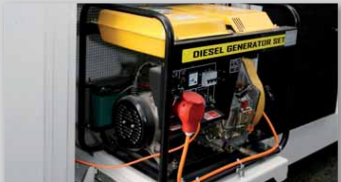
generator – easy fuelling by pulling it out to service/ fuelling position
