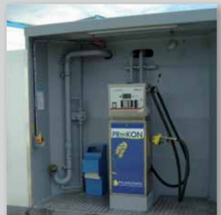
dispensing niche with gas pump; with standard equipment for vegetable oil; electrical niche, lockable, integrated in the front side of the container
