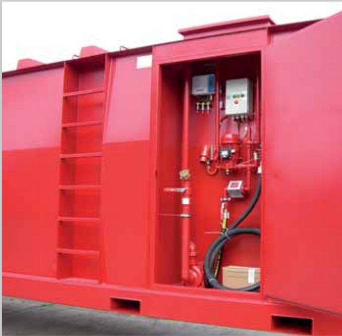
dispensing unit for 1 medium (diesel, biodiesel or gasoline)
