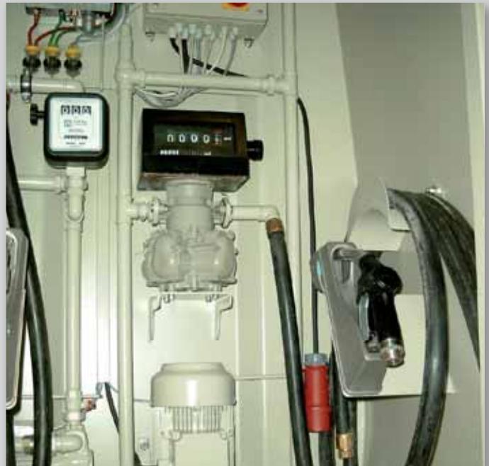
dispensing unit for 2 media (diesel, biodiesel or gasoline)
