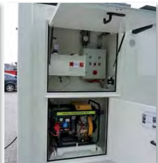
aggregate niche diesel generator, additional day tank, vacuum leak alarm device with system control and niche lighting
