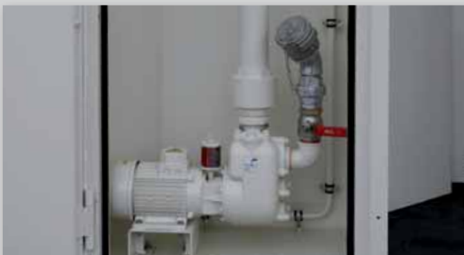
transfer pump for self-filling of the tank up to 1000 litre/min in lockable niche
