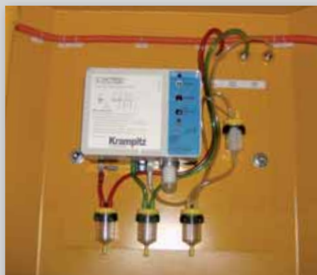
leak detecting device installed in the niche
